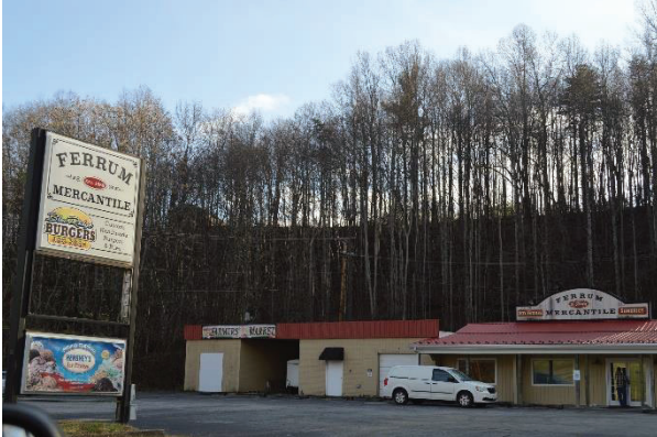
Photo 13: The Mercantile building is under redevelopment
