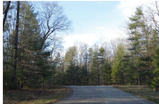
Figure 11: Franklin County built West Franklin Road to help prepare the site for private investment.
